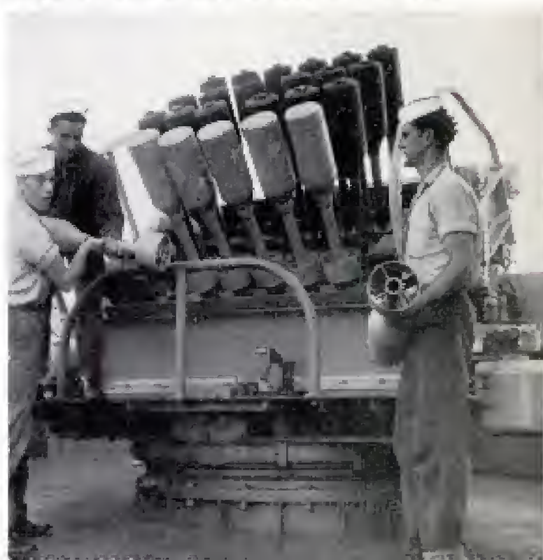
Sketch shows how surface ships make runs on midget sub T-2. Below, rocket-propelled "hedgehog" depth charges are launched singly, in series or all at once
